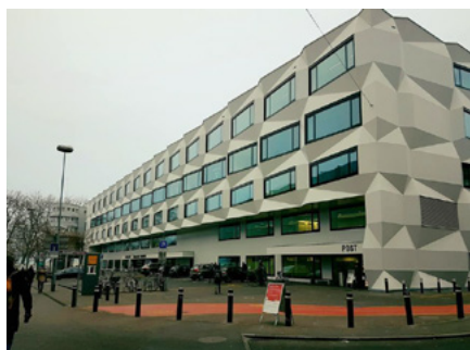
The new building of the University of Lucerne.
